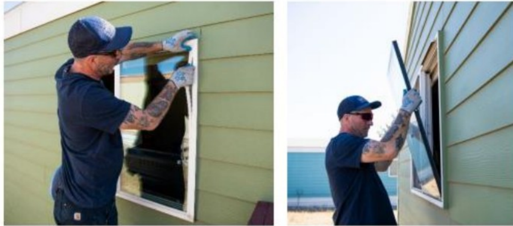
Figure 11. Thin triple-pane IGUs glazed into existing double-pane vinyl frames (Pasco, WA).
